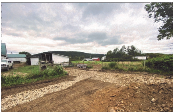
Figure 3. HUA after construction of diversion & subsurface drain.
