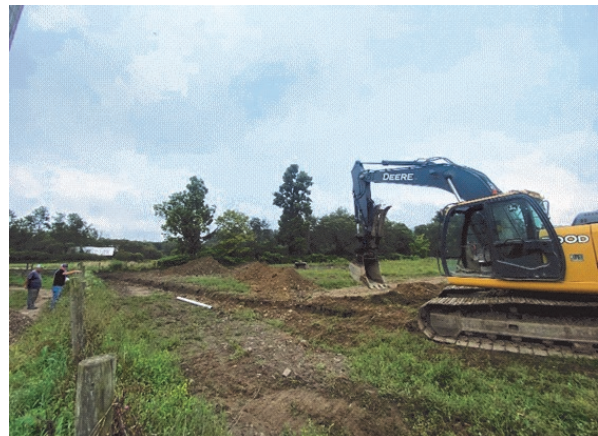
Figure 2. HUA during installation of subsurface drain.
